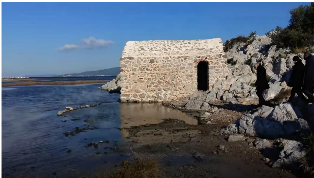
Figure 17. Disaster Risk Studies at IZTECH: Conservation of the Historic Geothermal Bath House in Gülbahçe, Izmir
